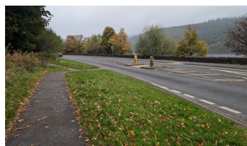
Ladybower Dam and 'plugholes' trail - main road crossing
