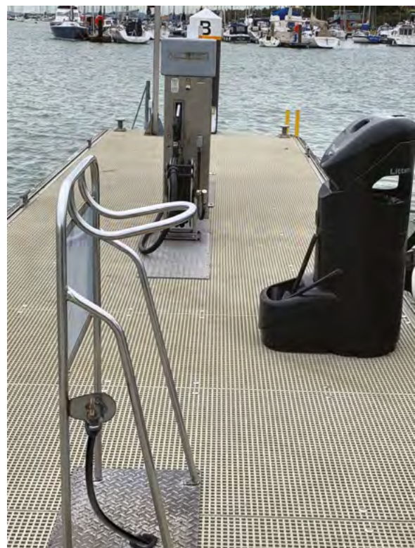
D. Fuel dock with HUT for hose use – with waterproof insulation removed
