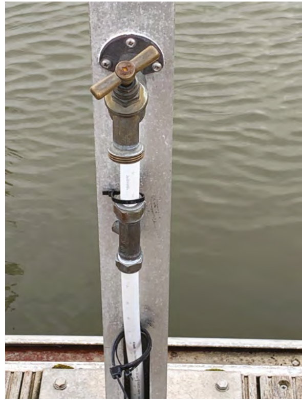
B. In-line suitably approved double check valve (DCV) – with waterproof insulation removed
