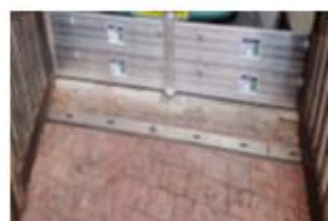
Garage barrier install
