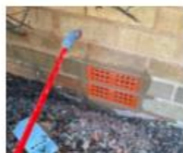
Air Brick Install
