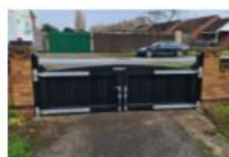
Double Flood Gates
