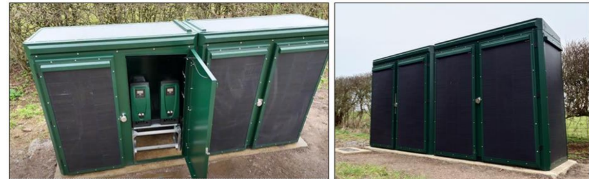
New pump and kiosk
