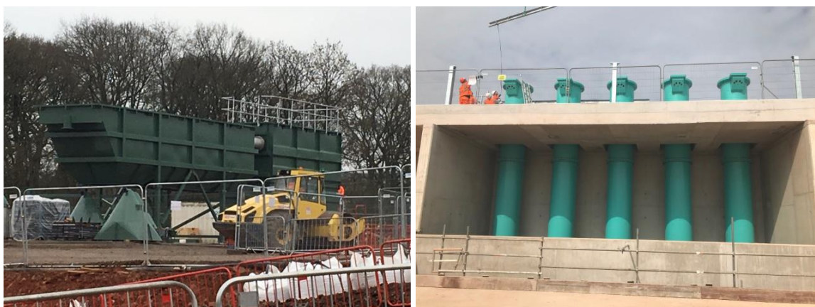
Plate: Installation of Sludge treatment Lamella no1. (March 2019) and Emergency Return Pumping Station ready for pump installation (April 2019)
