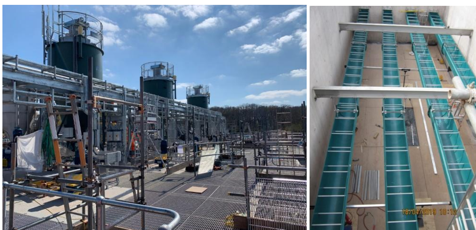
Plate: Progress on treatment process: View from SPL Actiflo clarifier roof and RGF outlet channels (April 2019)
