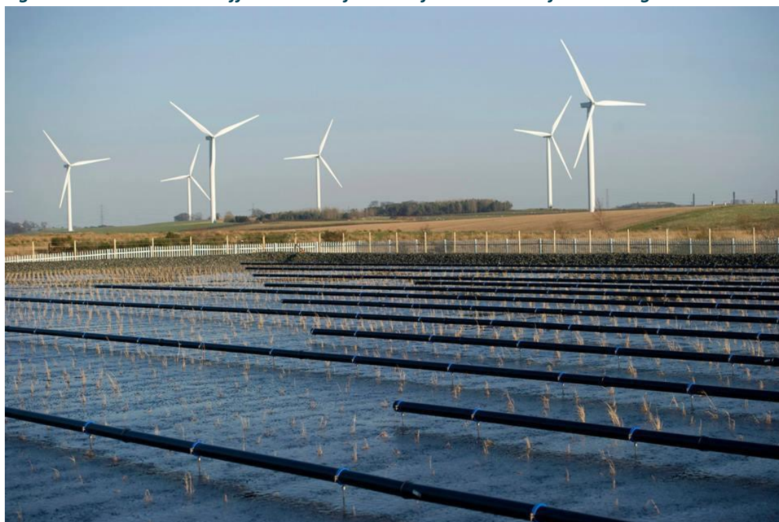
Figure 3: We will trial the effectiveness of vertical flow reed beds for reducing BOD levels
