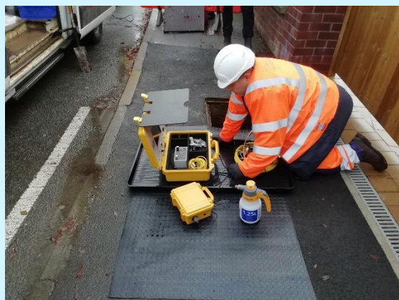
Figure 11: Micro-camera being used to review service pipe
