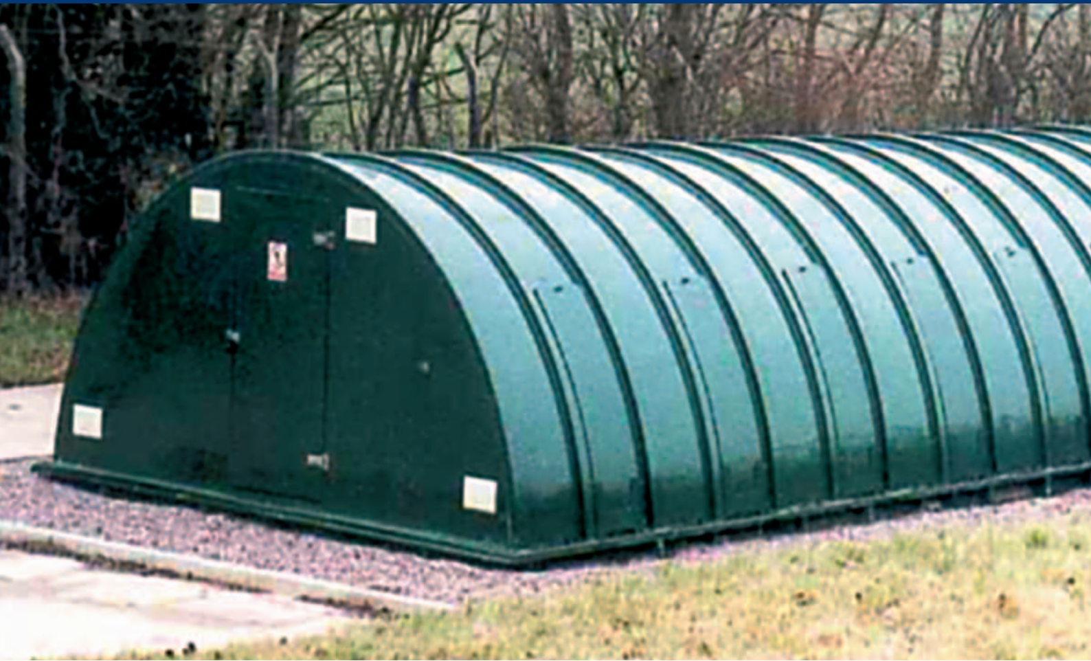
Rotating Biological Contactor (RBC)
