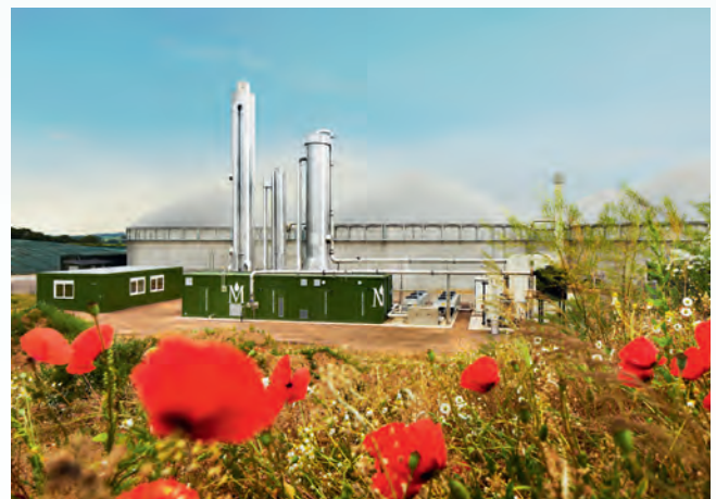
Returning energy to the national grid
