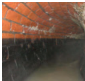
after cleaning the sewer
